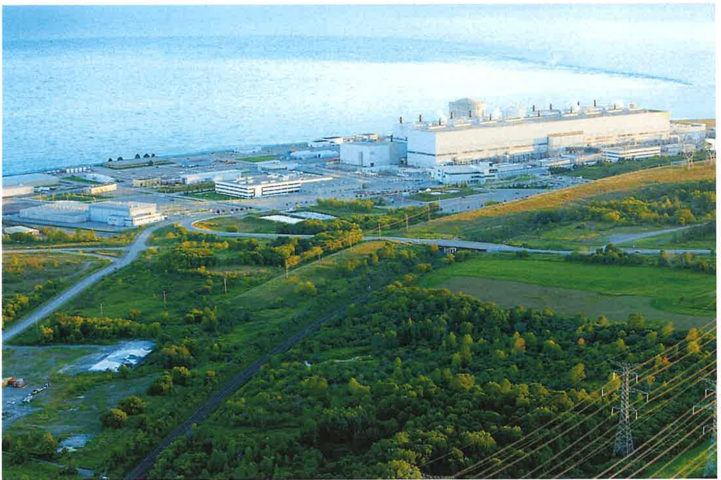
Darlington Nuclear Generating Station, Ontario SUPPLIED
